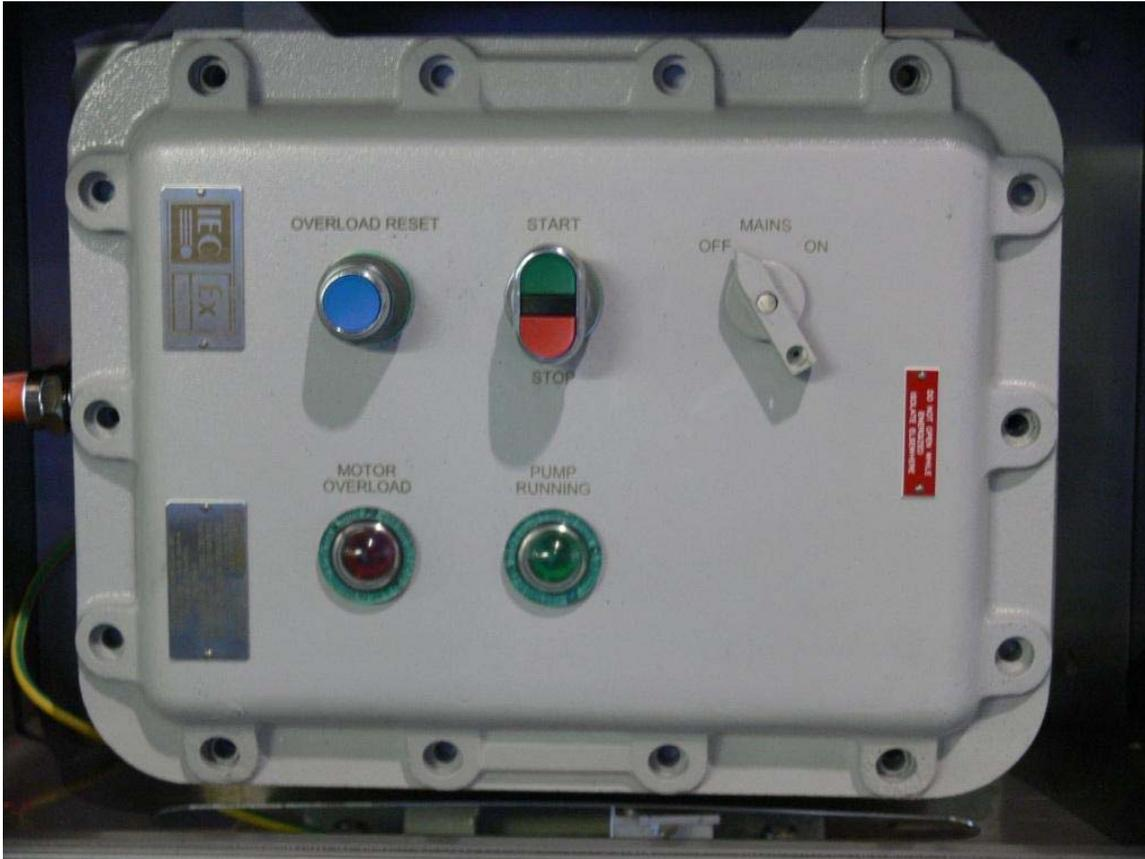
FJB432: an example of Ex d 15 kW star-delta motor starter with thermal overload and circuit breaker.
